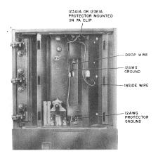
FIG. 5 - Protector Mounted in 2D-Type Set
