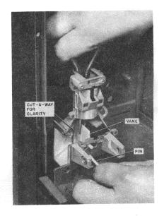
FIG. 4 — Installing Pin in Vane
